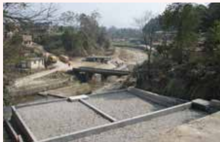
Polluted water refinery plant
